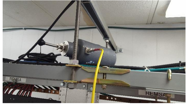
Motorola cavity filter in front of the Tek analyzer. The 10 dB BW was 10 MHz centered around 467.9 MHz
